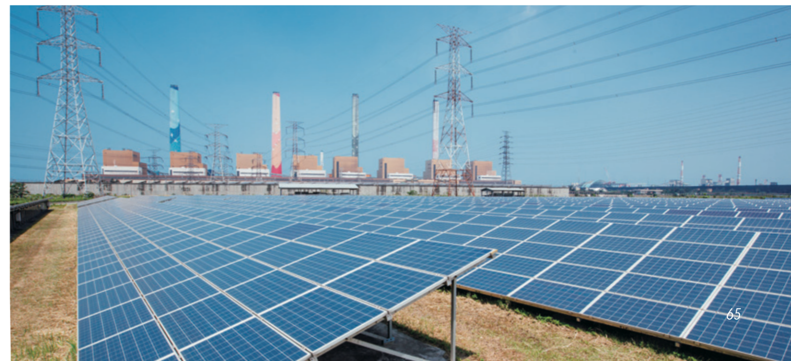
Longjing Solar Photovoltaic Field
