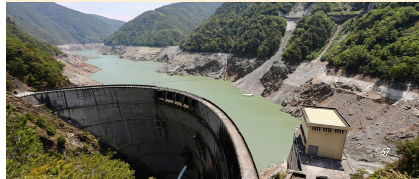
▼ Techii Dam dried up reservoir from water shortage
