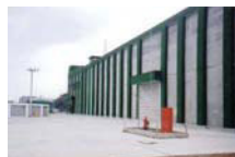
▶ The modern-day waste storage container at 1 st Nuclear Power Station
