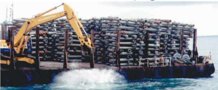
► Fish reefs made of electric poles.
