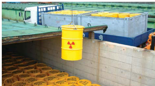
▶ Flasking solid low-radioactivity waste
