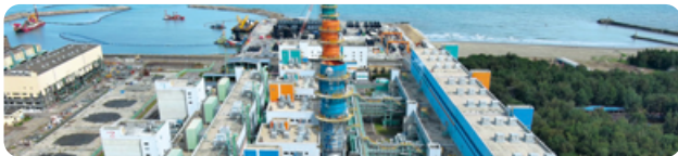
▲ The Tungshiao Power Plant is undergoing a major transformation, upgrading with expanded gas-fired power and moving forward with renewed momentum.
