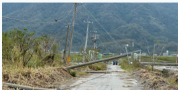
Damage in Hualien Caused by Typhoon Koinu
