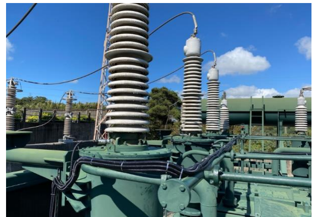
Figure 3. Sensor Wiring and Conduit Installation
