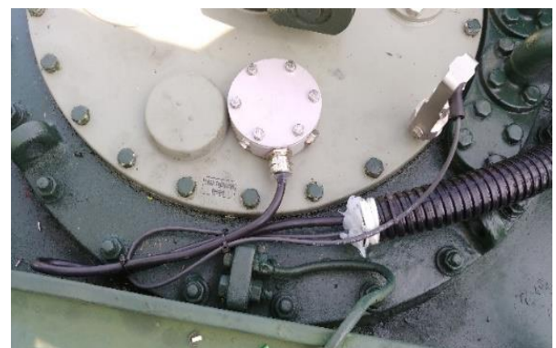
Figure 4. OLTC Monitoring Sensor and Cable Layout
