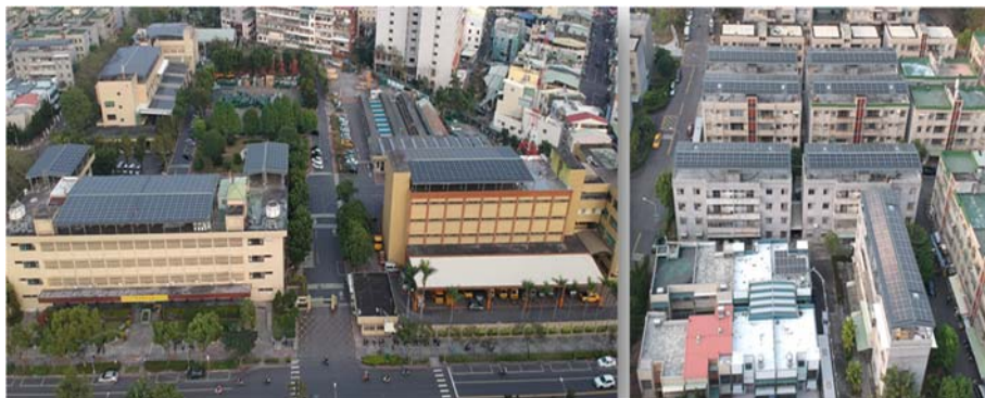
Figure 2 Photograph of 600kWp-PV(left) , Photograph of 200kWp-PV(right)
