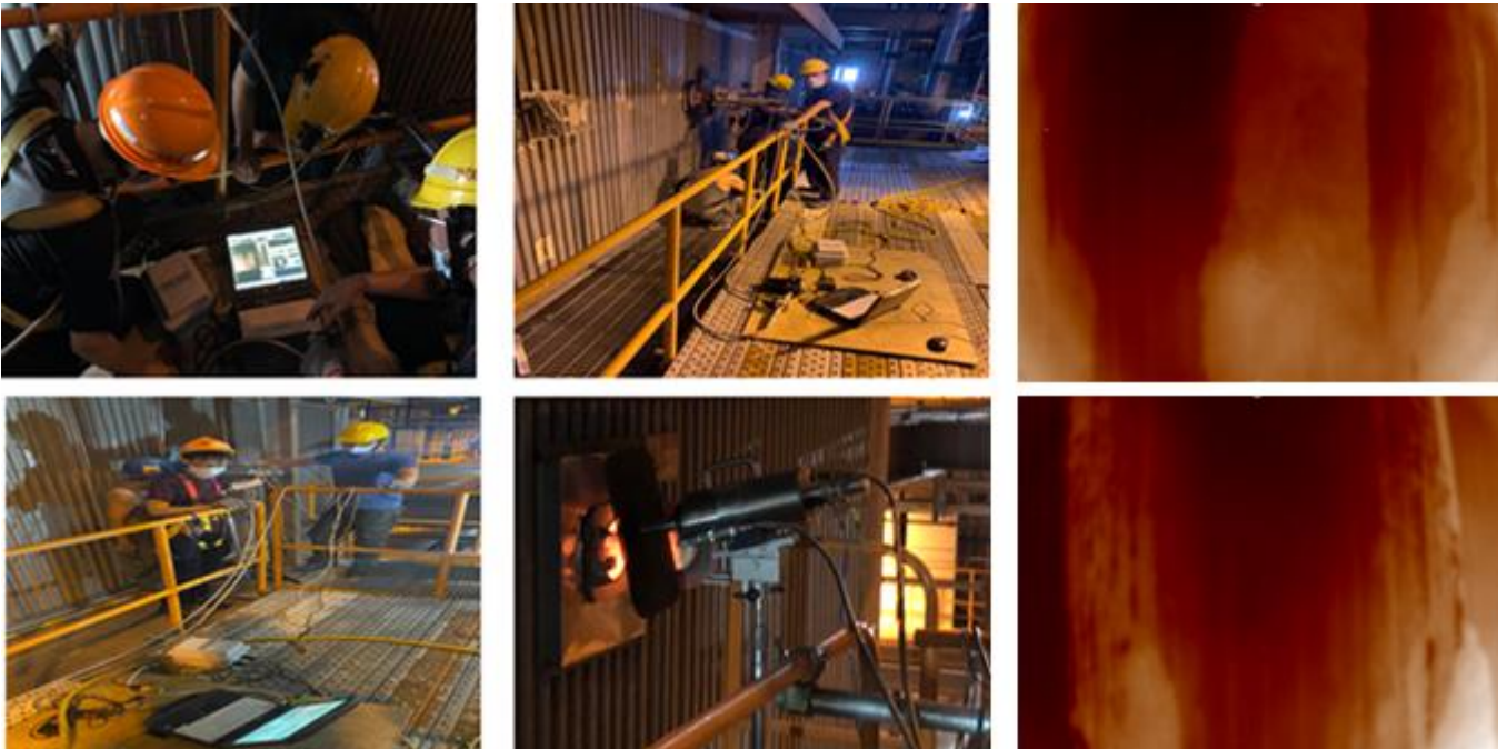
燃煤鍋爐過熱器線上結渣檢測 Online Slugging Monitoring of Superheaters in Coal-Fired Boilers
