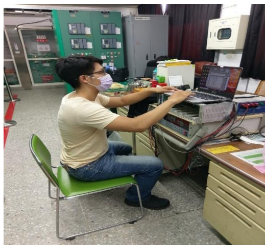
發電廠變電所監控儀表定期校驗 Regular calibration of monitoring instruments in power plant substations
