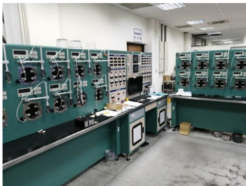
電度表修校自動化設備 Wathour Meter Repair Automation Equipment
