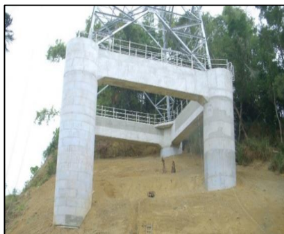
Figure 3 four-pile foundation structure
